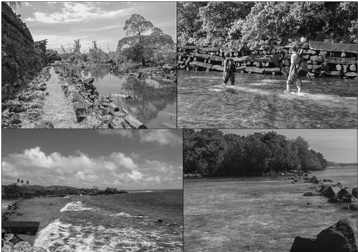
Figure 2. Nan Madol's artificial islets and breakwater walls. Clockwise from top left, examples of a canal, a path on top of an islet, and the outer face of the massive enclosing wall that rings Nan Dawas (H-113); a typical edge of an islet faced with columnar basalt stacked in the header-and-stretcher style; boulders aligned to create a breakwater wall; two parallel breakwater walls at Pahn Mwasangapw (H-128).
