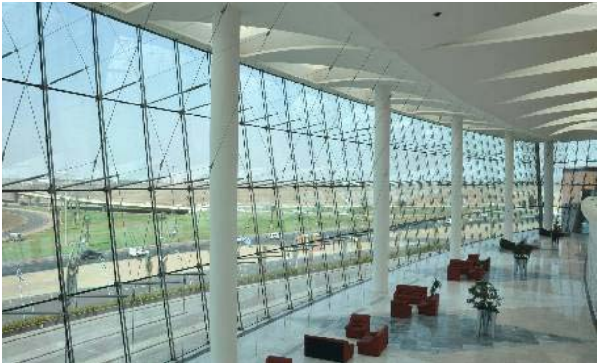
Mall of Arabia; Jeddah, Kingdom of Saudi Arabia Architect: ECHO Design; Riyadh / Kingdom of Saudi Arabia Facade Area: 5000 m 2 Facade construction with LOOP glass retaining ring and RODAN tie system
