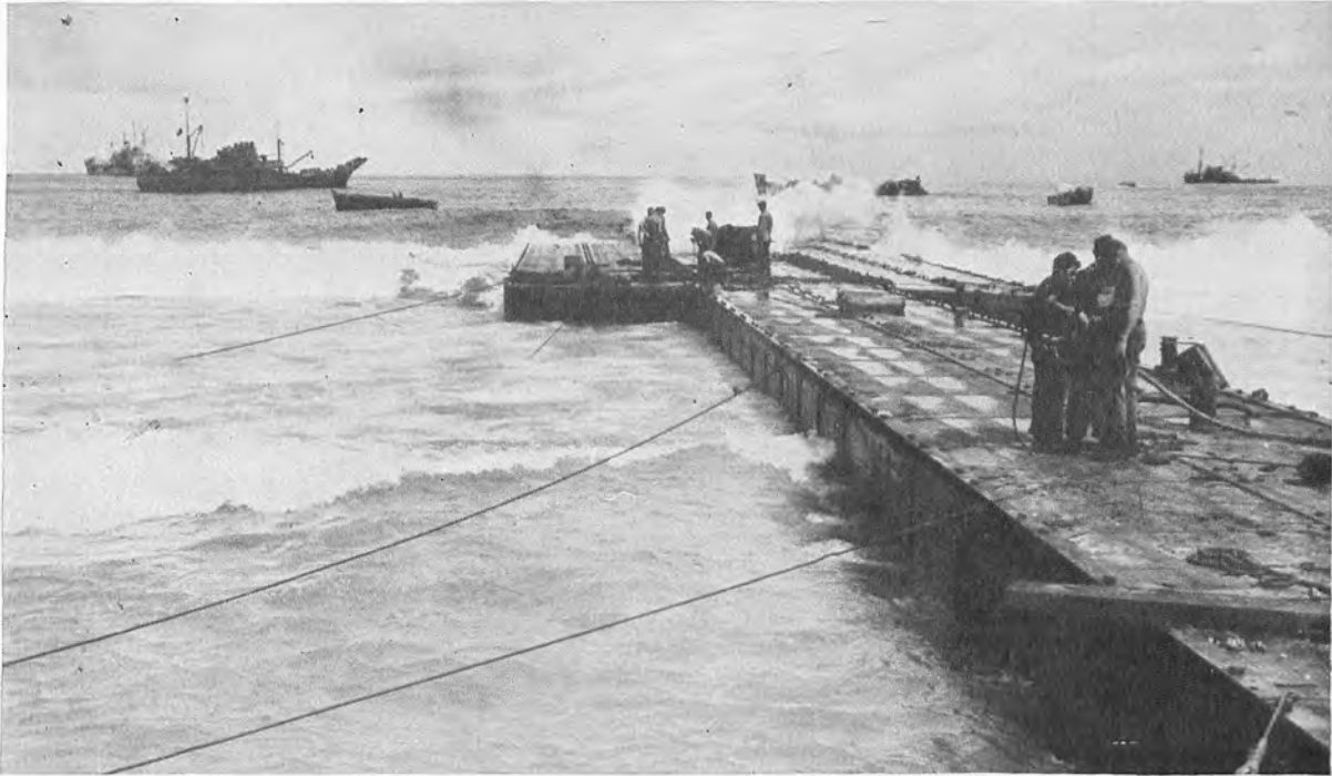
WHITE 2 CAUSEWAY , delayed in installation because of Japanese artillery fire, finally became operative on the afternoon of Jig-plus 3 (27 July). This prefabricated pier and the one at White 1 enabled LST's, LCT's, and LCM's to pull alongside and unload cargo. Unfortunately, the causeways had a short life, both being wrecked by the storm on the night of 29-30 July.
