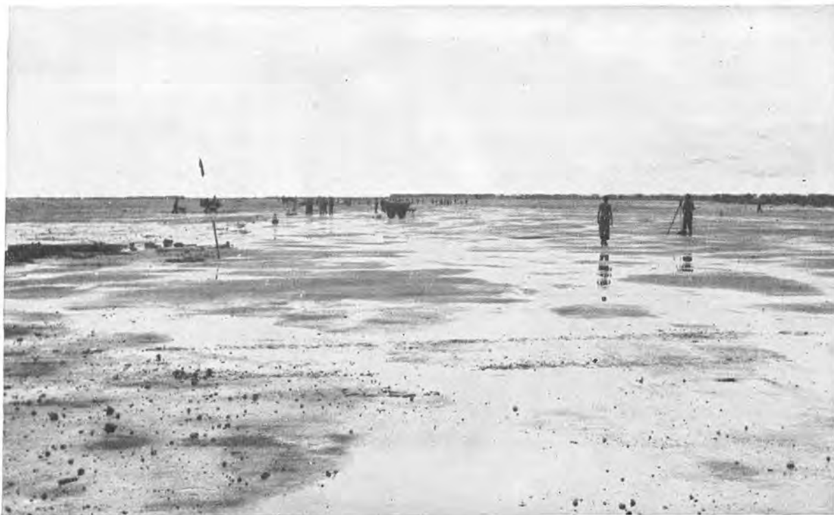
USHI POINT AIRFIELD , wet from one of Tinian's frequent downpours. Since relatively little of the U. S. preparatory bombardment was directed against the field, damage to it was minor. By 29 July the strip extended 4,700 feet in a single, hard-surfaced runway.
