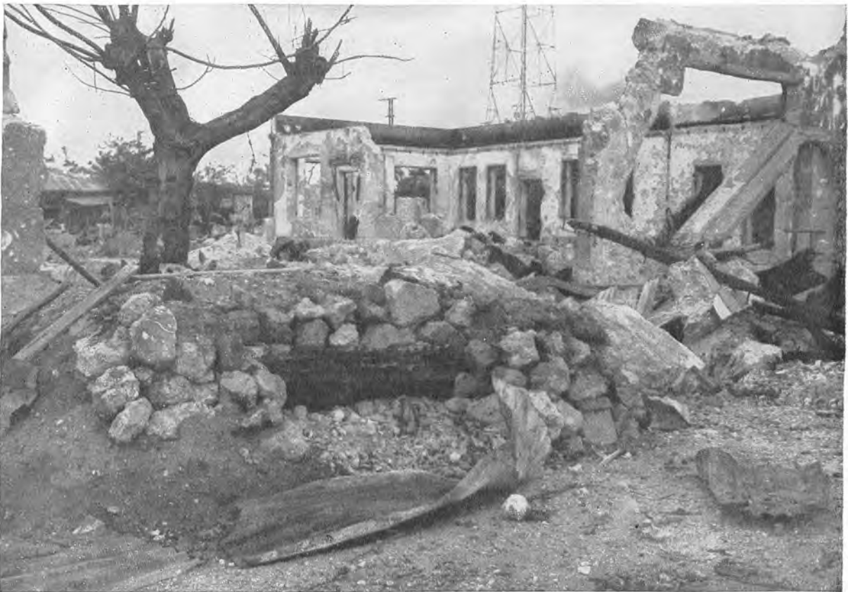
MACHINE-GUN POSITION in the center of Tinian Town was well-constructed, well-sited, and, fortunately for the Marines, unoccupied. No dead and only one live Japanese remained in the town on 30 July.
