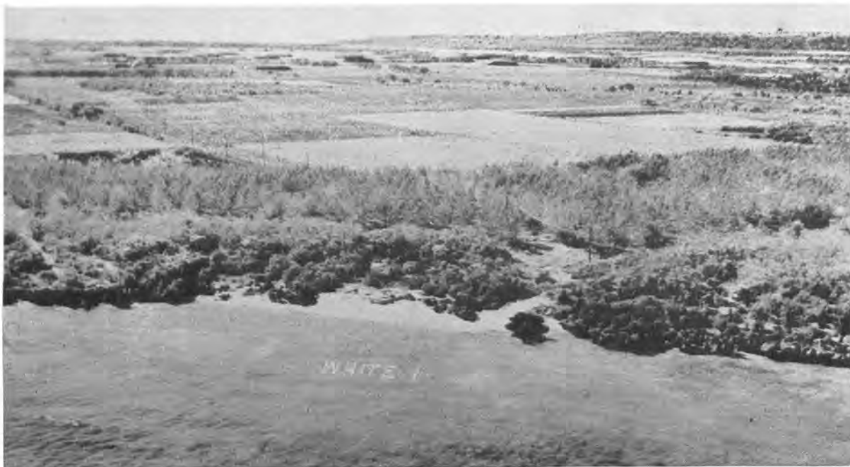
WHITE 1 BEFORE naval gunfire, artillery, air and bulldozers altered its appearance. This 60-yard beach later became the port of entry for most of the V Corps' heavy equipment.
