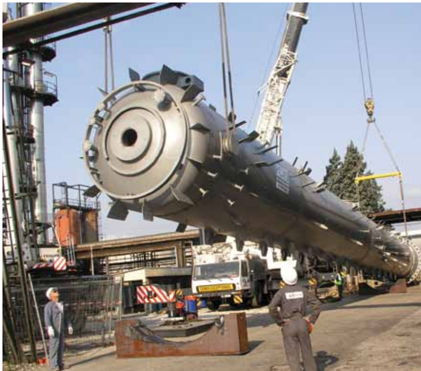
Installation of an industrial ECR type column on site
