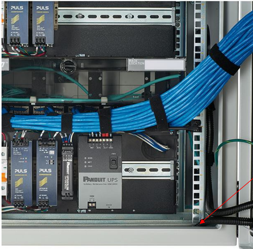
Figure 12 - Routing power cable across the hinge and through the duct
