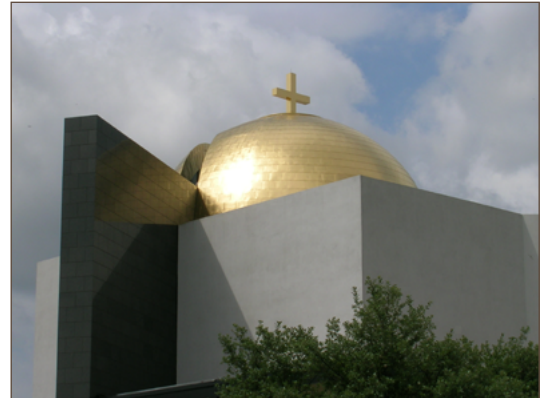
Figure 3.3C. Gilded copper dome crowns the Chapel of St. Basil in Houston, Texas; Niko Contracting, sheet metal installer.
