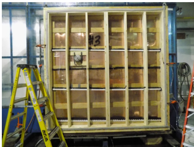
Figure 15.6.2: Vertical copper double lock standing seam. View from inside face of wall assembly during ASTM E331 water penetration test.
