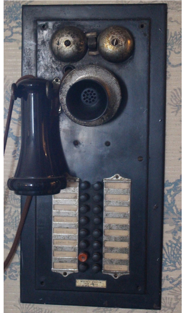
Communication system in Servants' Hall
