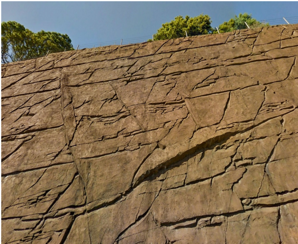
Photo 3 – Sculpted Wall Facing without Joints
