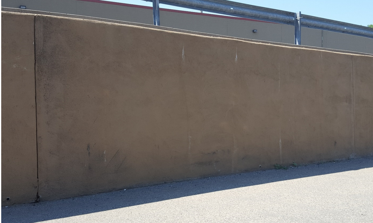
Photo 6- Expansion Joint on the Left and Contraction Joint on the Right
