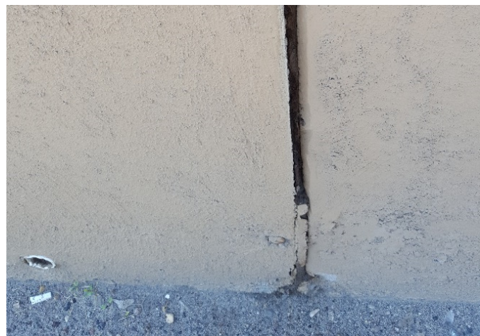
Photo 5 – Expansion Joint and Detail
