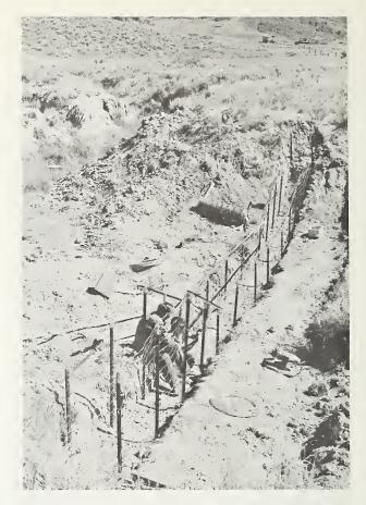
Figure 27.—Parallel fences for double-fence dam (see fig. 11) are being installed. Note the excavations for key, apron, and bank protection (the latter two to right of the structure).
