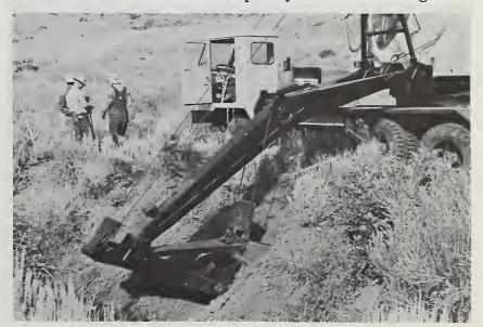
Figure 25.—The key for a rock check dam is efficiently excavated with a backhoe.
