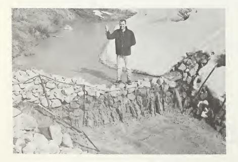
Figure 19.—Because this doublefence rock check dam was built with an insufficient portion of small rocks, many large voids allow water jets through the structure. Note that water is not running over the spillway. The jets endanger the stability of the structural keys and bank protection work. was estimated not to exceed  $0.75 \text{ m}^3$ /s, the 31- to 45-cm size class could be eliminated and 55 percent of the volume could be in the 20- to 30-cm class.
