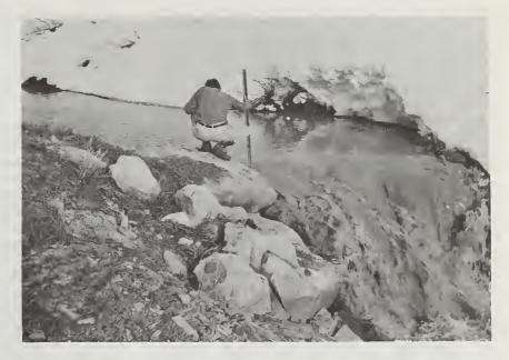
Figure 23.—Upstream view of a loose-rock check dam supporting a discharge of about 0.3 m<sup>3</sup>/s. Effective dam height is 1.7 m.
