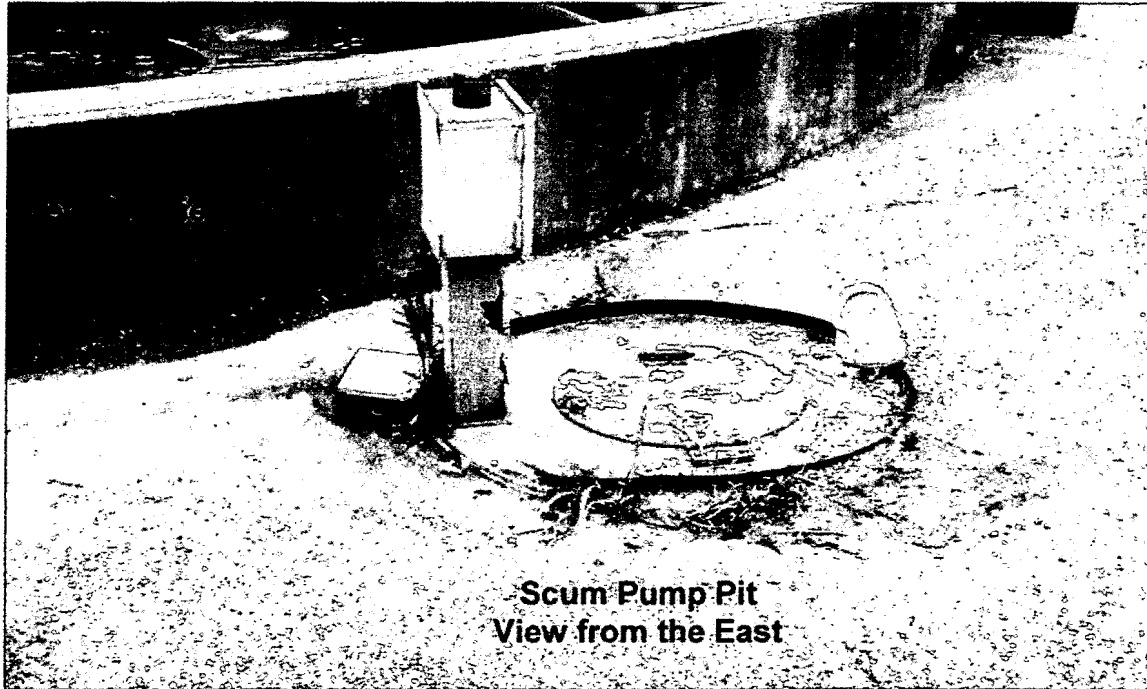
MWWTP Building/Structures Before Demolition
