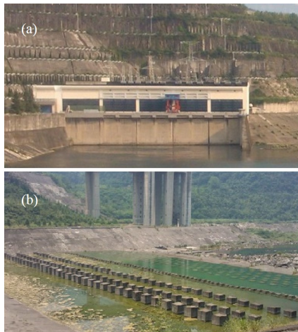
Figure 4. Linear structural targets in the dam area: (a) power plant; (b) stilling pool in water retaining wall.
